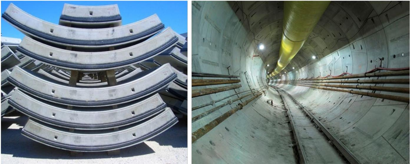
Figure 10.21 Precast Concrete Tunnel Lining
