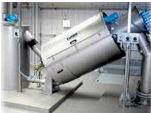
**Figure 8-7 Rotary Screw Thickener (Courtesy of Huber)**
