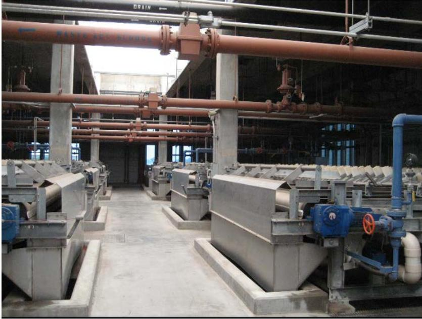
**Figure 8-5** Installed Gravity Belt Thickeners at the Bissell WWTP
