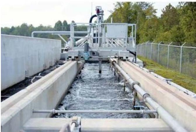
Figure 3-1 Grit Removal Channel
