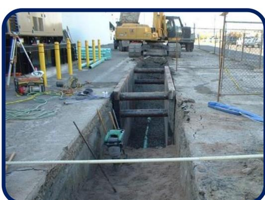
New sewer segment #3 will be constructed via open excavation within the existing easement
