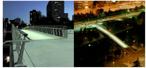
**Figure 121:** Cork Town Pedestrian Bridge: Soft light floods the bridge floor from glare free LED lighting in the handrail, allowing safe use of the bridge without trespass to the low light level landscape below.
