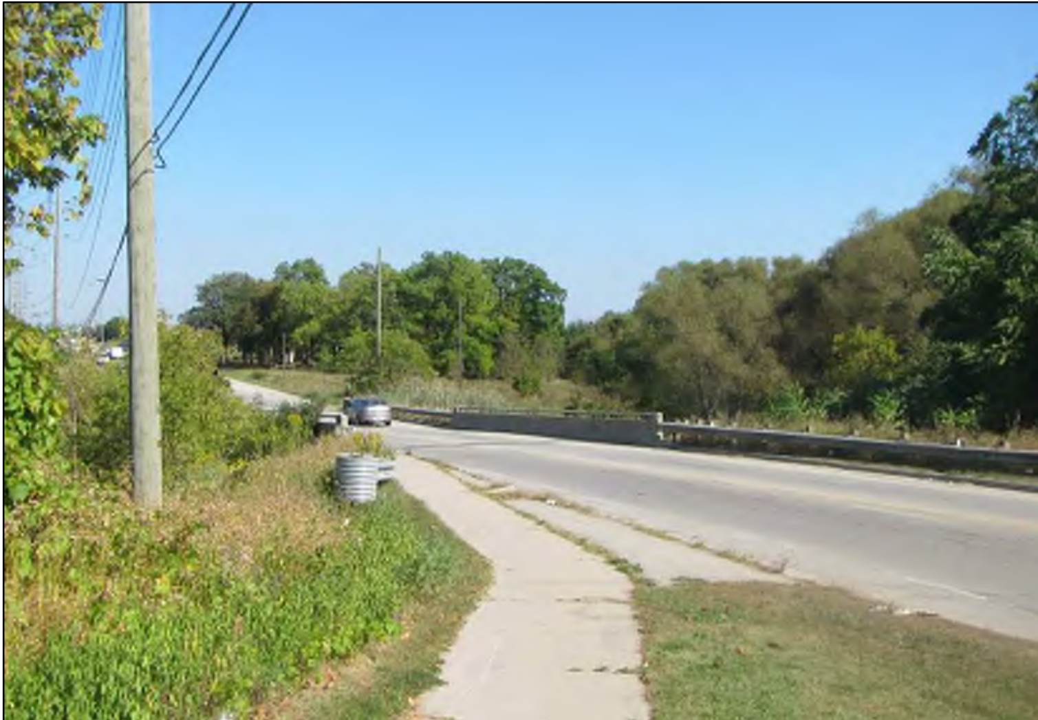
Photograph 24: Existing Langstaff Avenue bridge over the West Don River, looking southeast (September 21, 2017).
