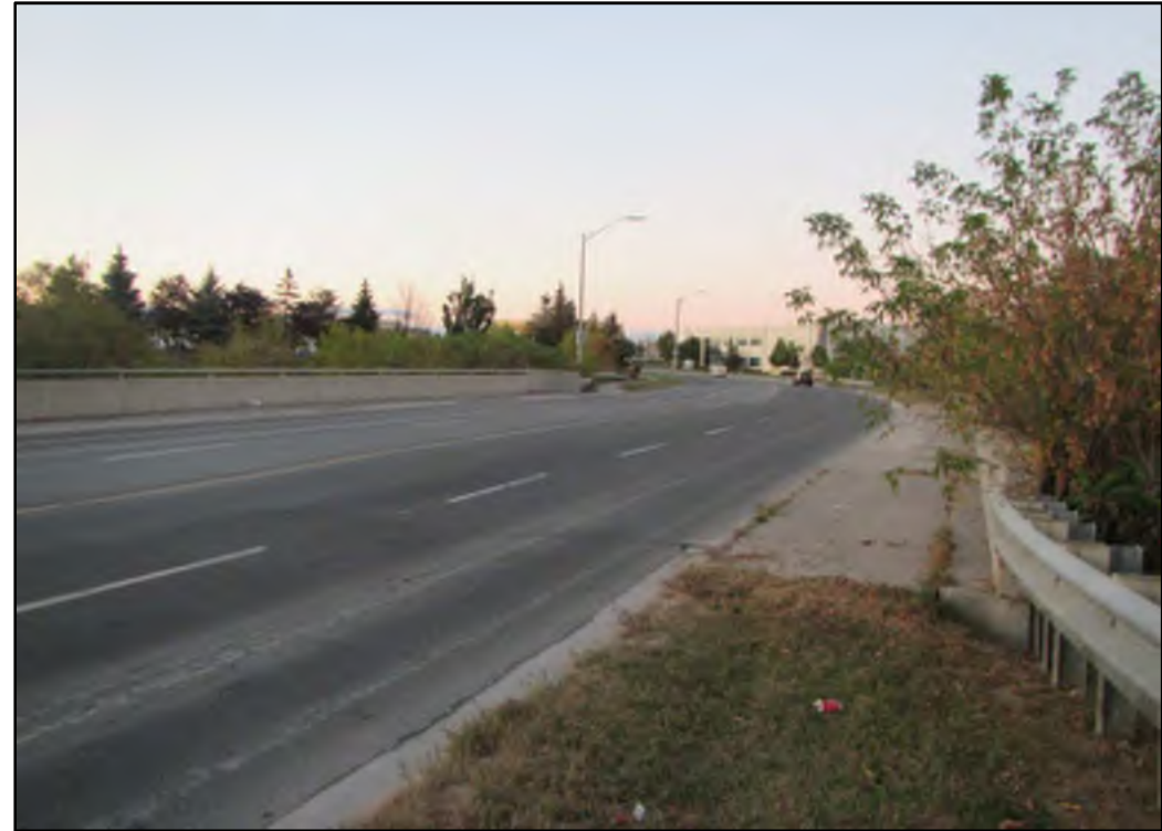
Photograph 18: Creditstone Bridge over the West Don River, looking north (September 28, 2017).
