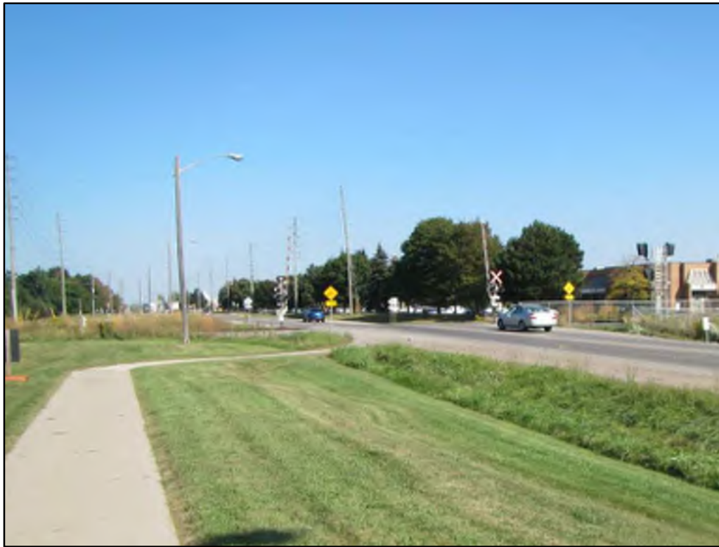
Photograph 33: Existing level railroad crossing of Langstaff Road and the Metrolinx Railroad, looking east (September 21, 2017).
