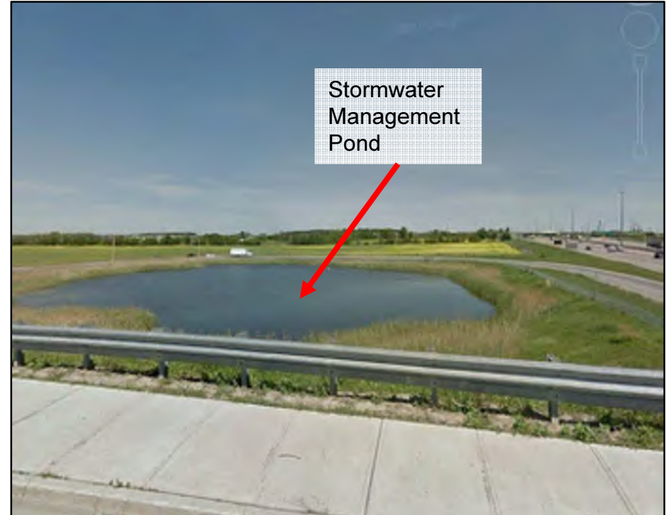
Photograph 9: Stormwater management pond within interchange loop from Bass Pro Mills Drive to Highway 400 W-S Ramp. Source: Google Street View.
