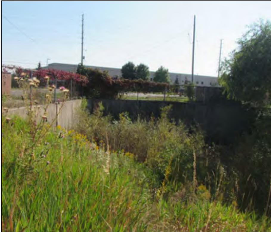
Photograph 39: Westminster Creek culvert, north side of Langstaff Road (September 21, 2017).
