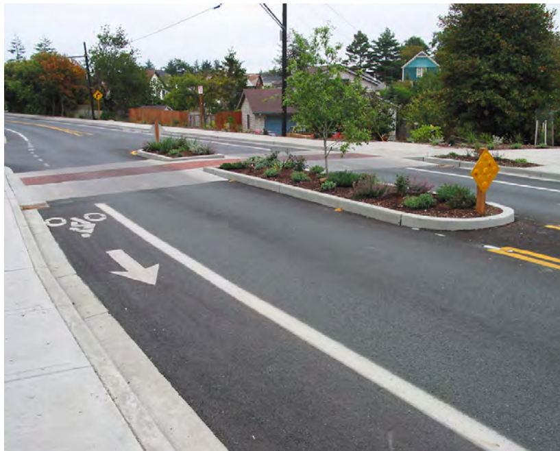
Figure 33. Midblock raised crossing with refuge island
