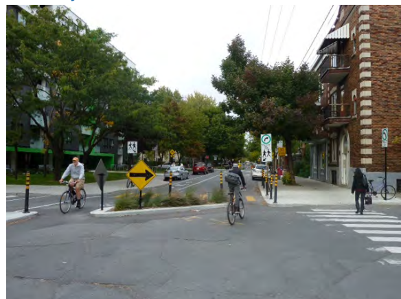
Figure 22. A diverter with selective filtration near an elementary school on Gilford Street in Montreal
