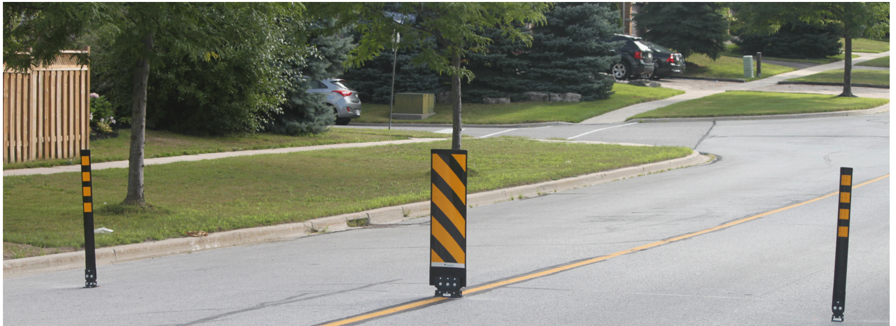
Figure 21. Choke point created with flexible bollards (Newmarket, ON)
