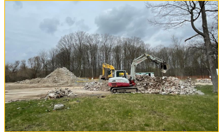
Image above: photo of demolition
