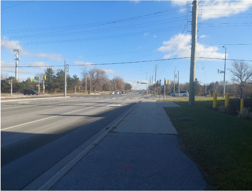
Plate 18: Major Mackenzie Drive, looking east towards Kennedy Road.
