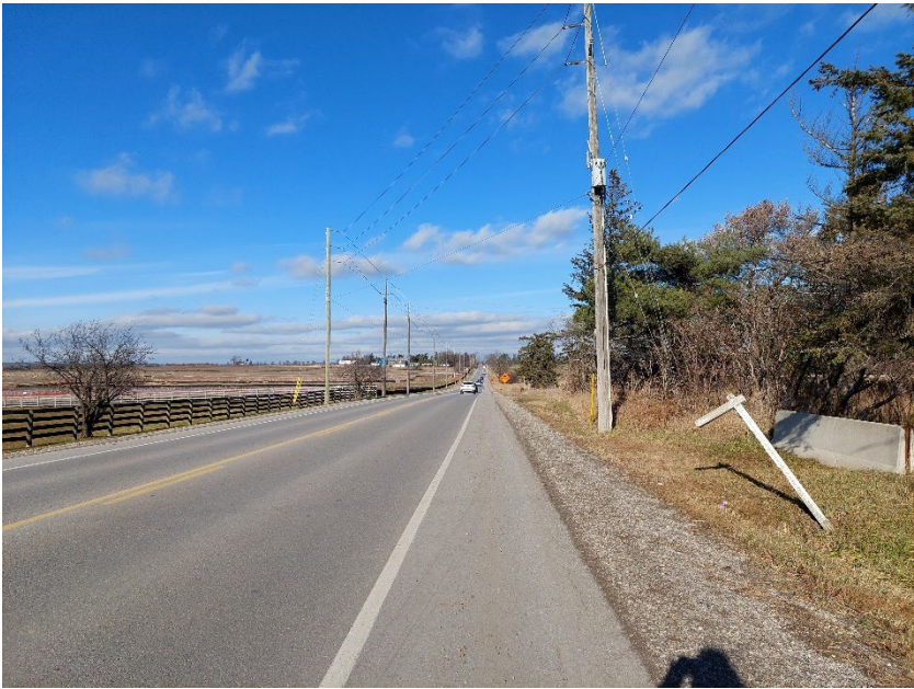
Plate 3: View north along Warden Avenue. The roadway now lacks curbs and sidewalks.
