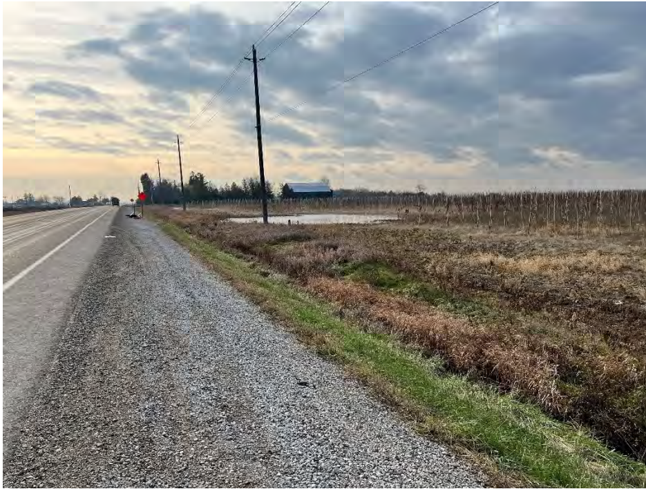
Image 20: Kennedy Road, road right-of-way is disturbed, no potential. Property beyond has potential, requires Stage 2 survey.
