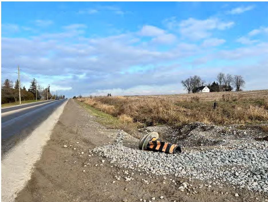
Image 14: Kennedy Road, road right-of-way is disturbed, no potential. Property beyond has potential, requires Stage 2 survey.
