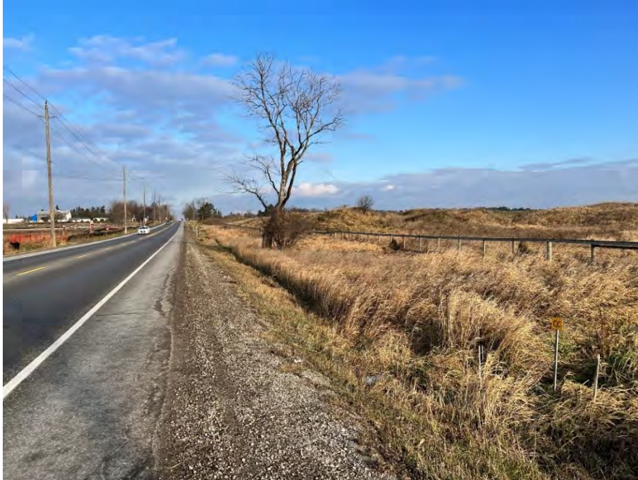
Image 6: Warden Avenue, roadbed and ditch is disturbed. Lands above ditch have potential, require Stage 2 survey. Culvert in foreground leads to low and wet area, no potential.
