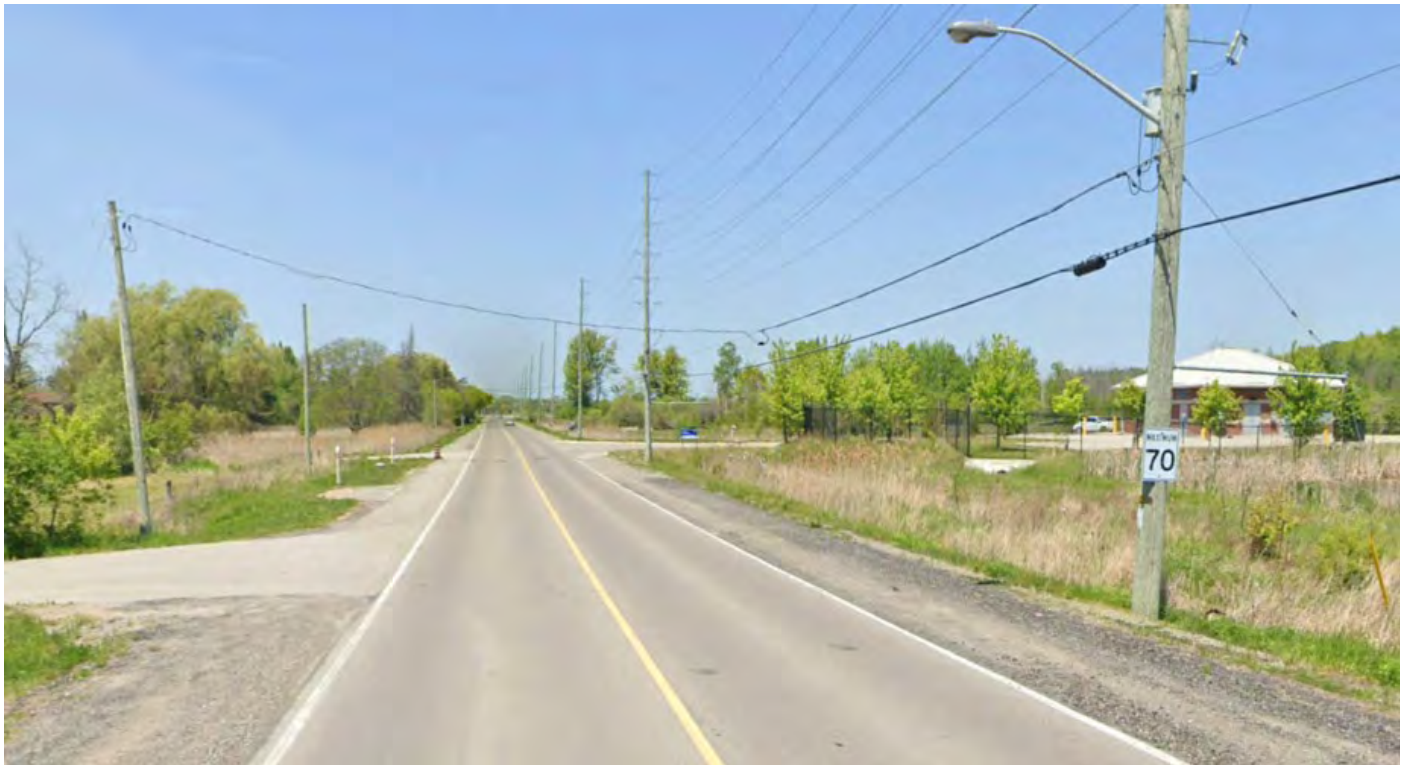
Figure 4.9 2nd Concession Road Looking North Towards Existing Queensville SPS and Queensville Sideroad. (Google Maps "Streetview," digital images http://maps.google.com )
