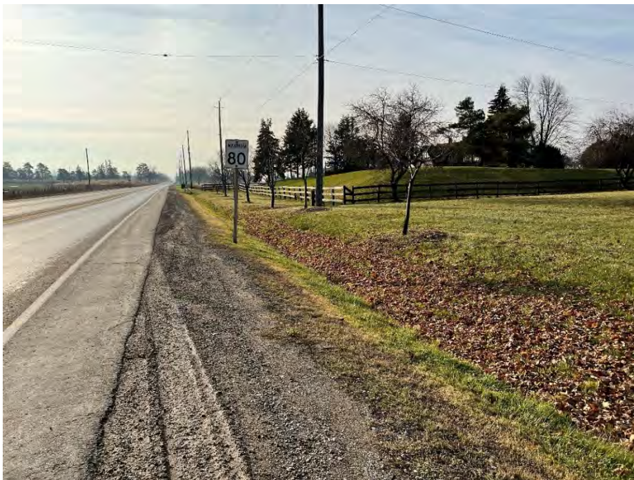
Image 11: Warden Avenue, roadbed and ditch is disturbed. Lands above ditch have potential, require Stage 2 survey. Raised berm in the background is disturbed, no potential.
