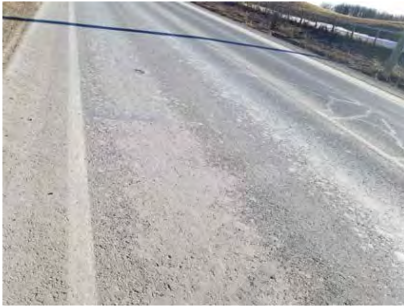
Section 2 – Asphalt surface near the construction site
