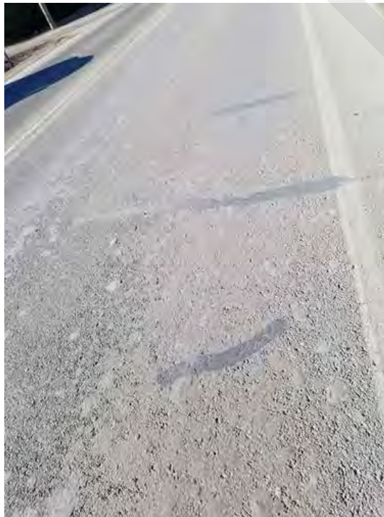
Section 2 – Asphalt surface near the construction site
