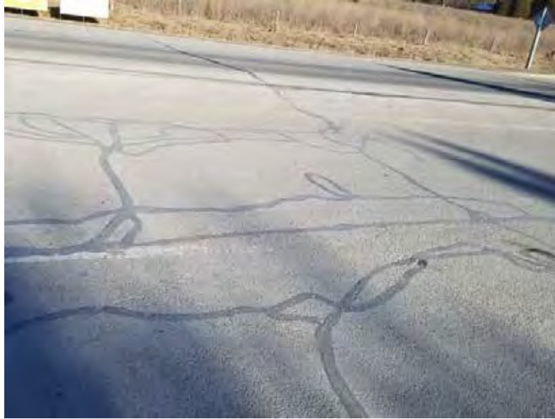
Section 2 – Sealed cracks
