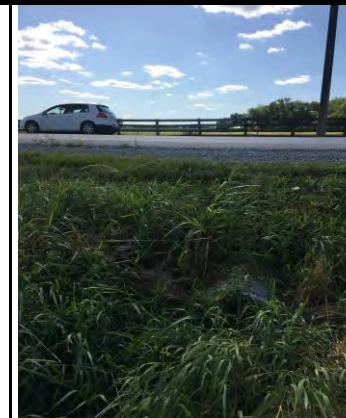
Downstream Structure Face
