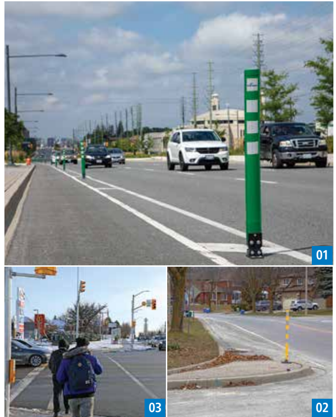
▲ PHOTOS (Top left and clockwise): 01 Bollards on the road separating the roadway from the cycle path. 02 A curb extension that improves pedestrian visibility 03 Leading pedestrian intervals that give pedestrians a head start at an intersection.
