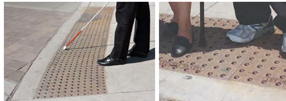
Figure 210 & 211: Accessible Exterior Routes And Curb Ramps Contribute to a Vibrant Streetscape.
