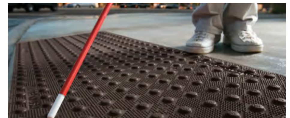
Figure 213: Tactile Attention Surface Indicators Located at Curb Ramps
