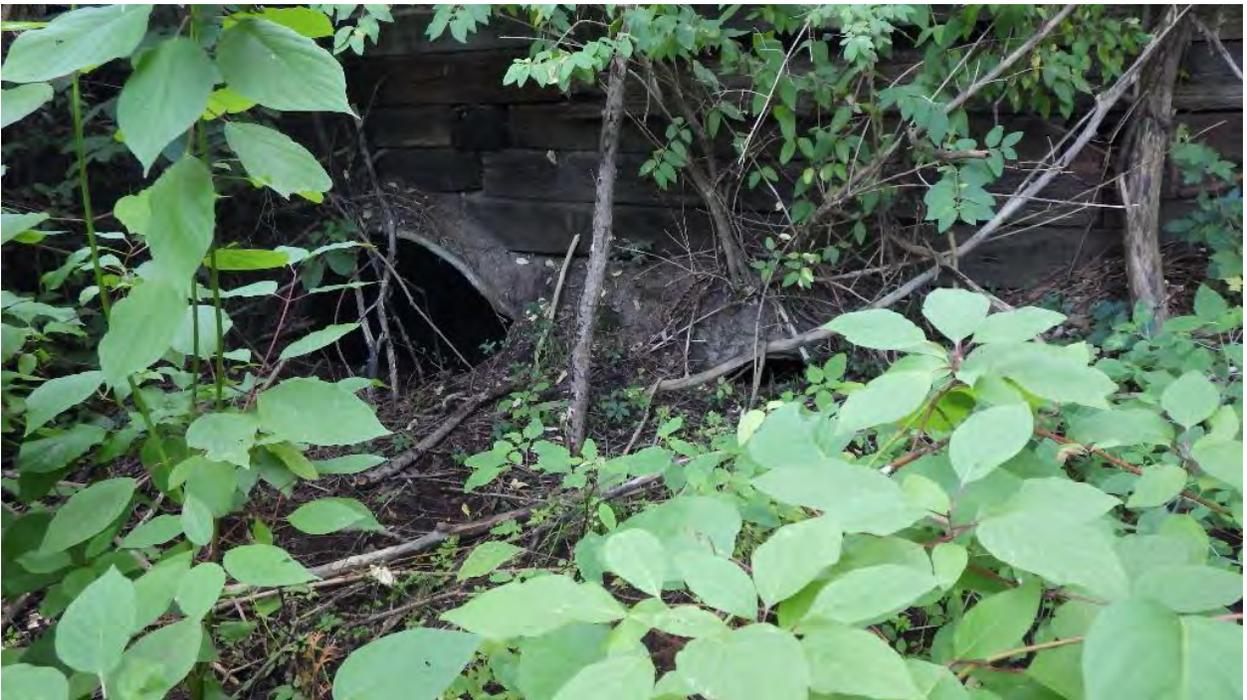
Photo 14: Fisheries Site 2 - Pedestrian bridge on private property with blocked CSP culverts
