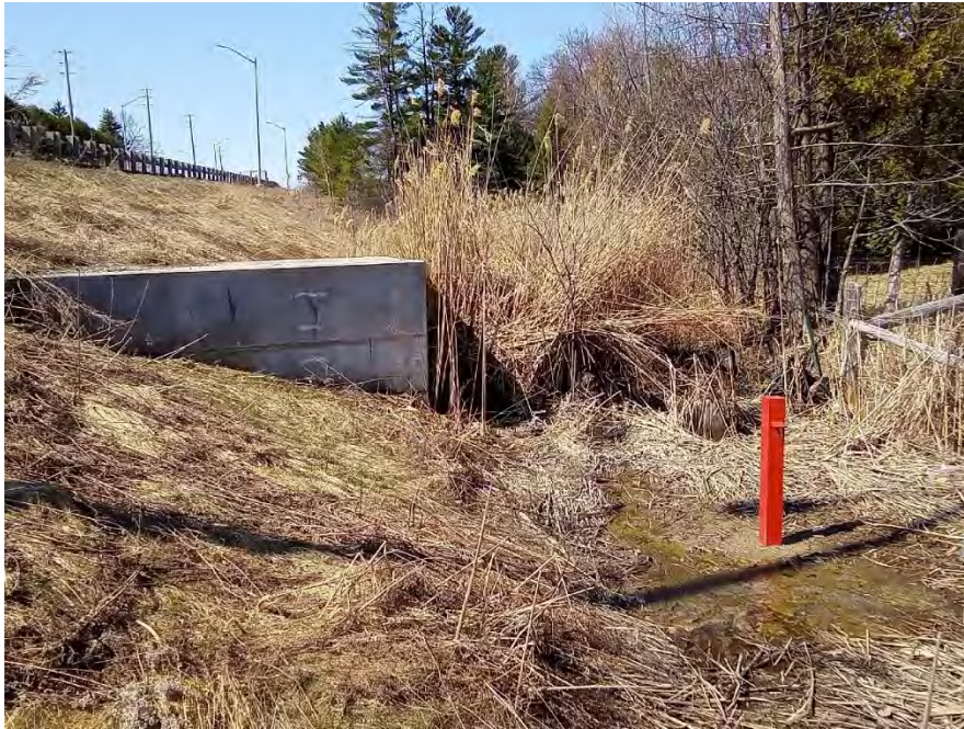
Image 37: Disturbed Teston Road right-of-way and channelized creek; no potential.
