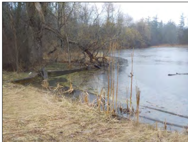
Photo 2: Dam creating the in-line pond and delineating the reach break
