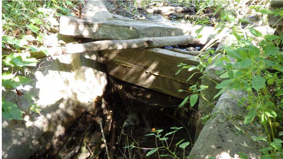
Figure 2 – Existing Dam at Pond Outlet
