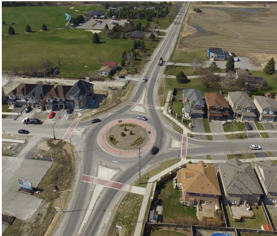
Figure 3 Ninth Line and Bayberry Street
