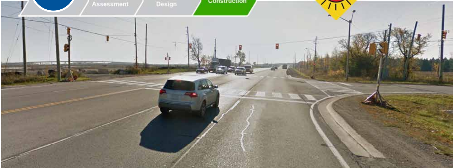
Intersection improvements including northbound double left-turn lanes
