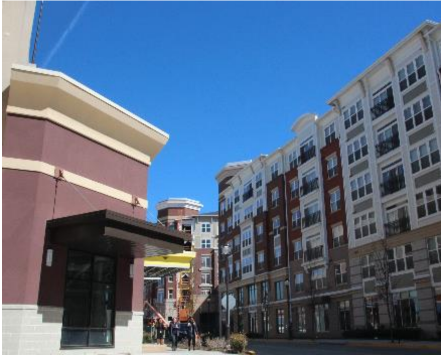
Former Park-Ride Lot Dunn Loring Metro Station Vienna, Virginia
