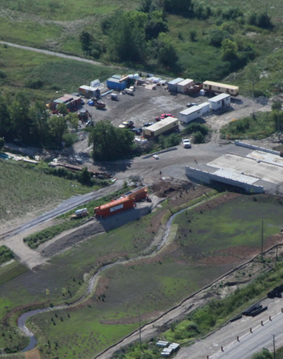
Bayview Avenue – Watercourse Relocation and New Structure
