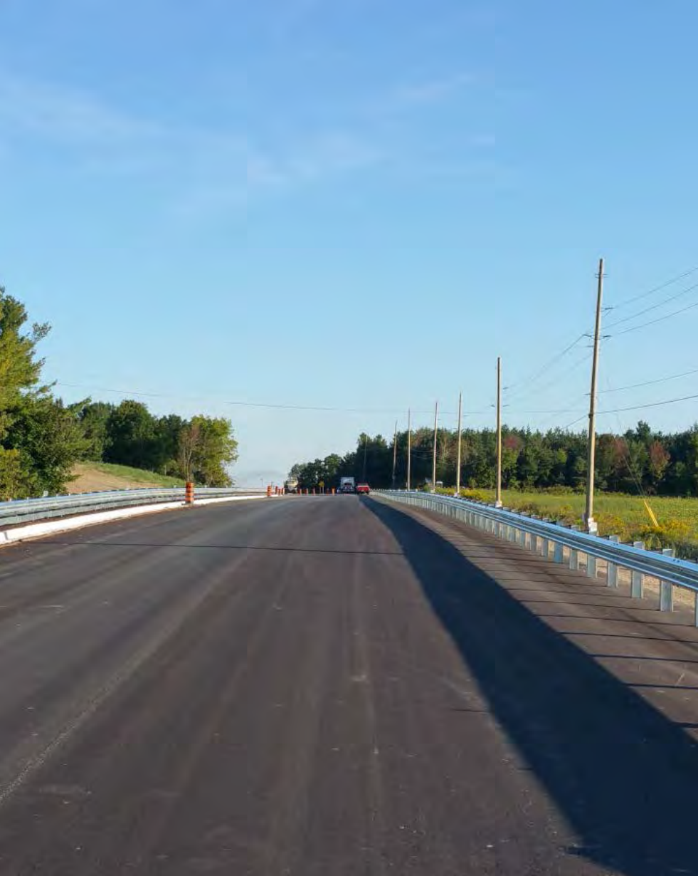
Bathurst Street – Road Paved and Guiderails Installed
