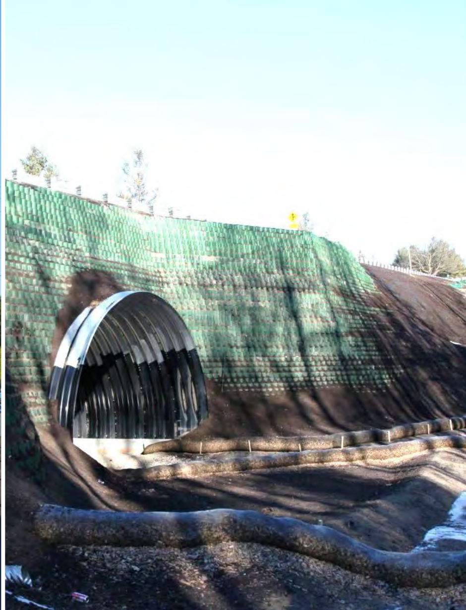
Bathurst Street – Culvert
