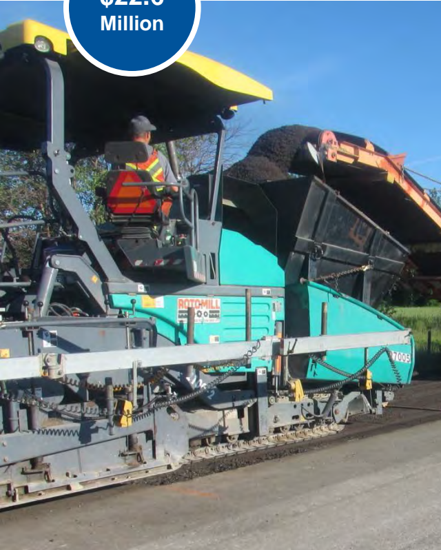
Road Rehabilitation and Preservation
