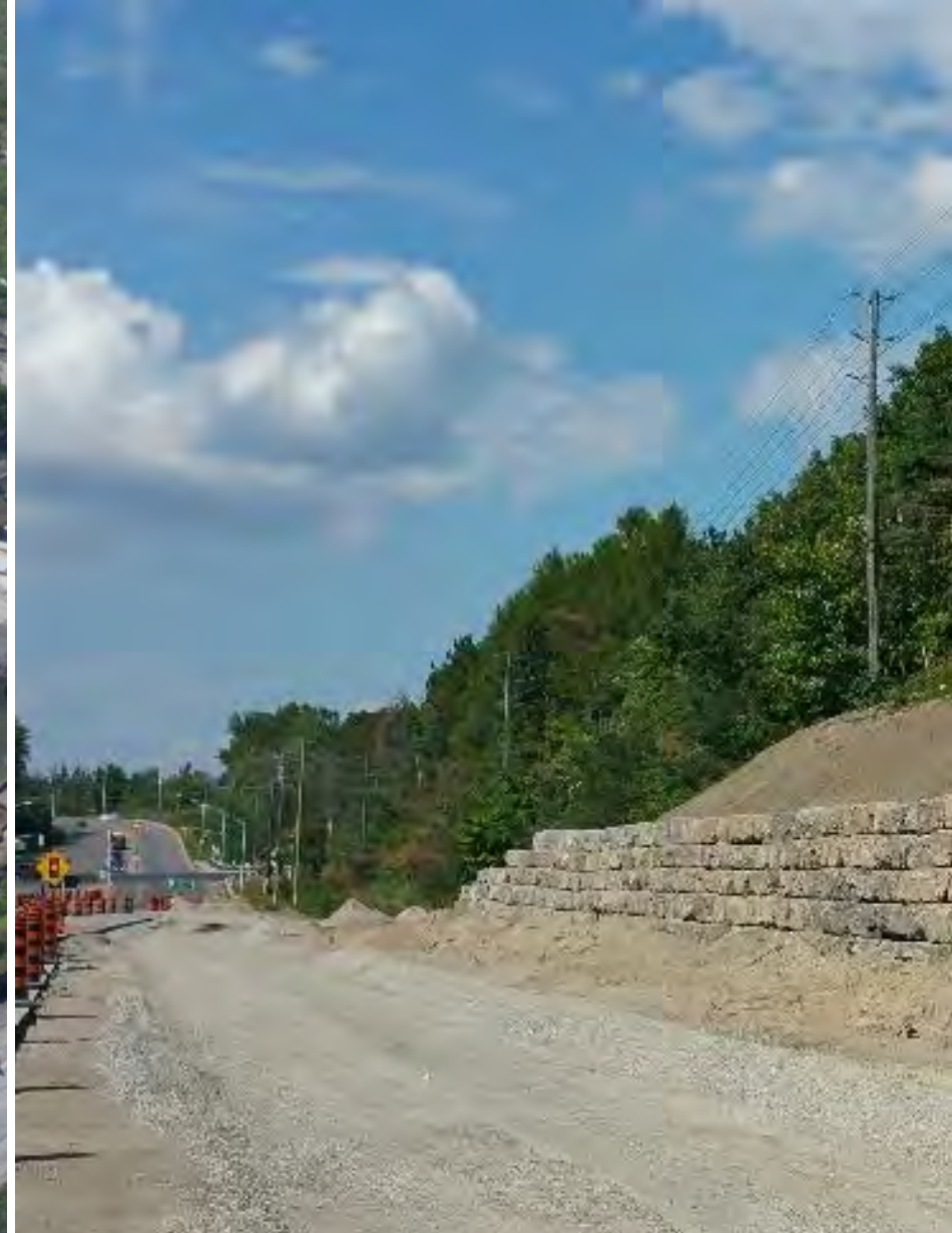
Bayview Avenue – Retaining Wall
