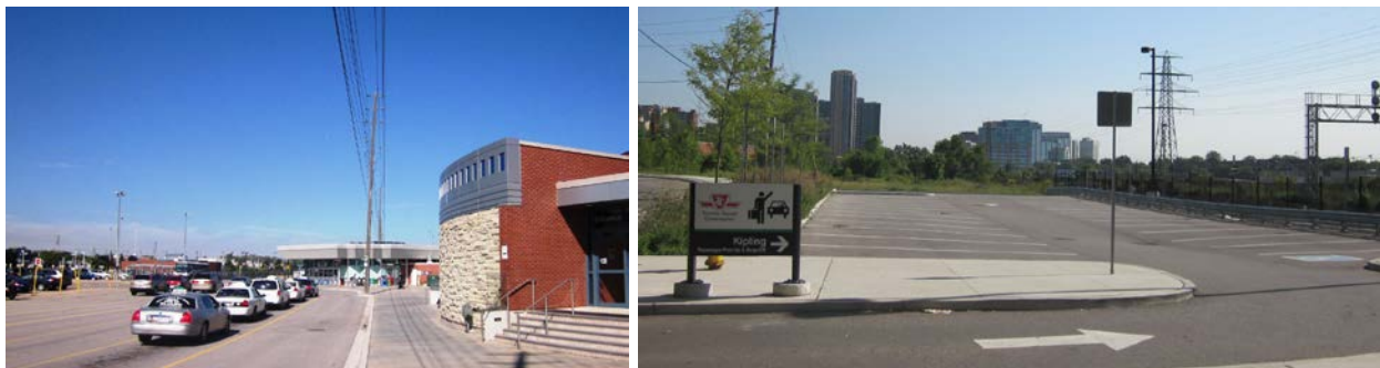
Figure 6: LEFT – Current queuing-style of PUDO with taxi lane at Oakville GO/VIA Station. RIGHT – Short term parking style of PUDO at Kipling TTC east station entrance.
