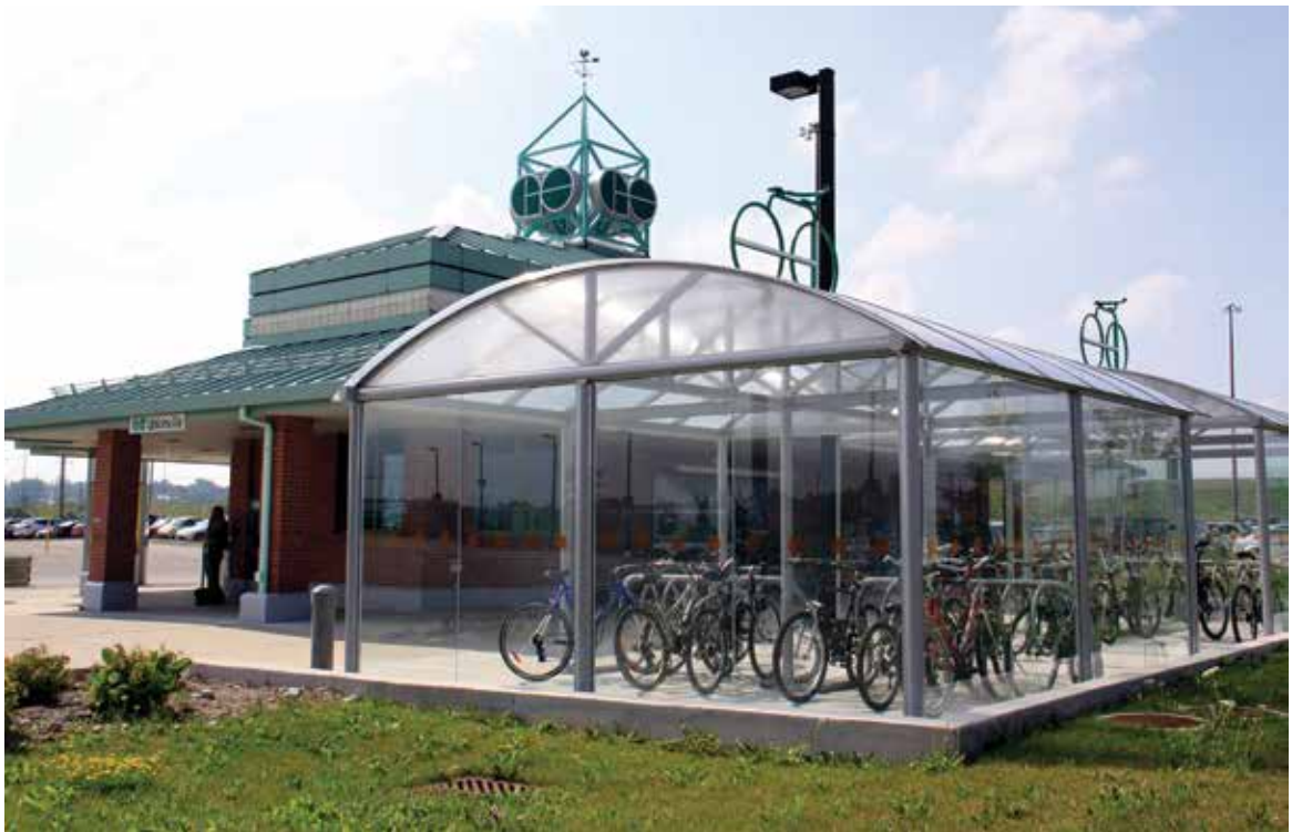
Unionville GO train station parking lot and bicycle parking in the City of Markham
