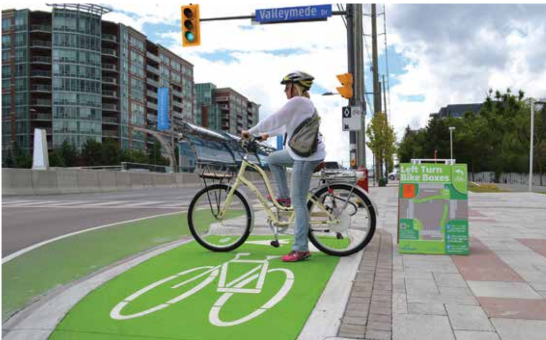
In-boulevard green colour treatment left turn bike box on Highway 7
