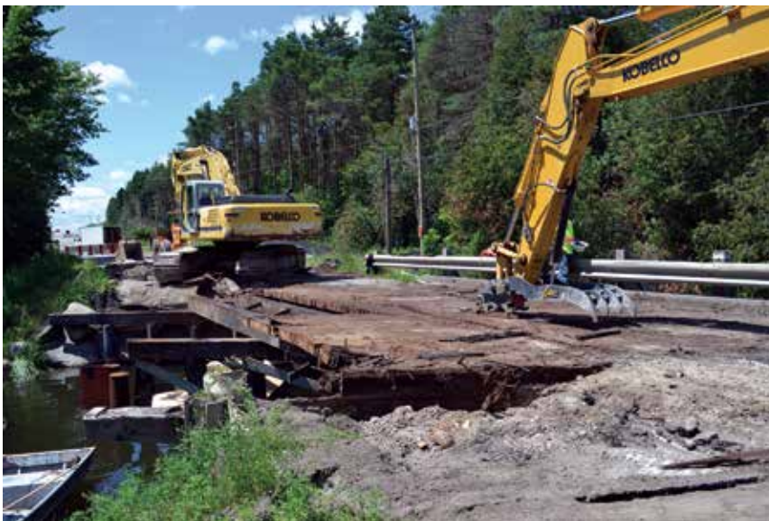
Umphrey Bridge rehabilitation
