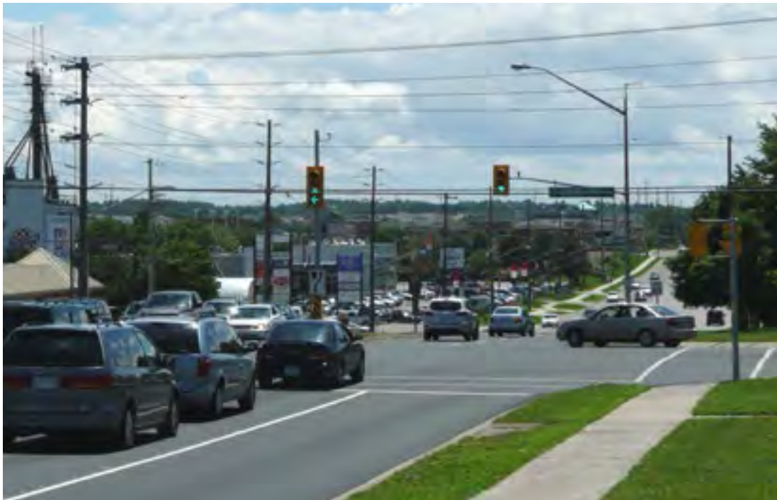
A Signalized Intersection in the Town of Newmarket
