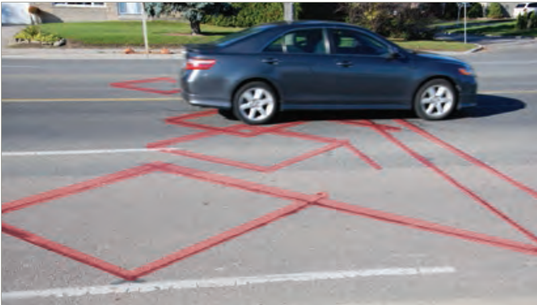
Example of permanent count station for cars, trucks and buses (Leslie Street, south of Queensville Sideroad).
