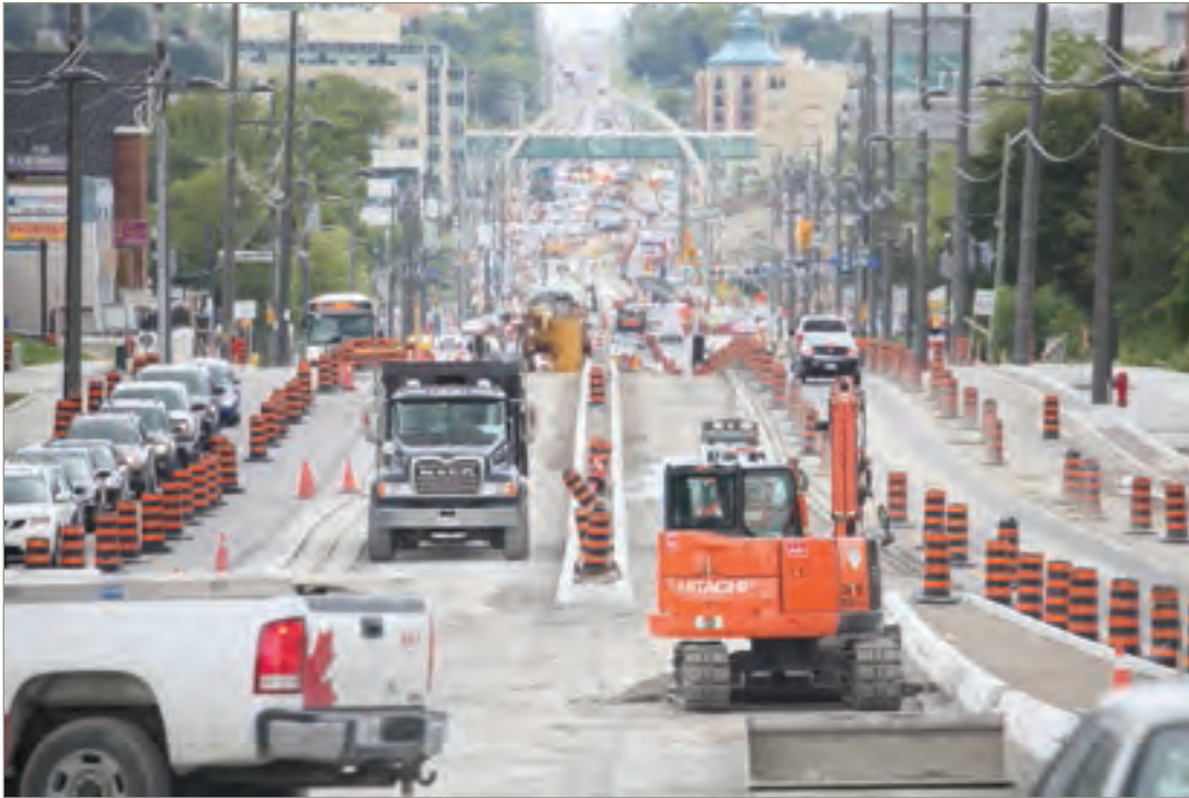
VivaNext construction on Davis Drive in the Town of Newmarket
