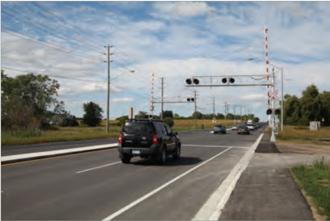
At-grade railway crossing in the City of Markham
