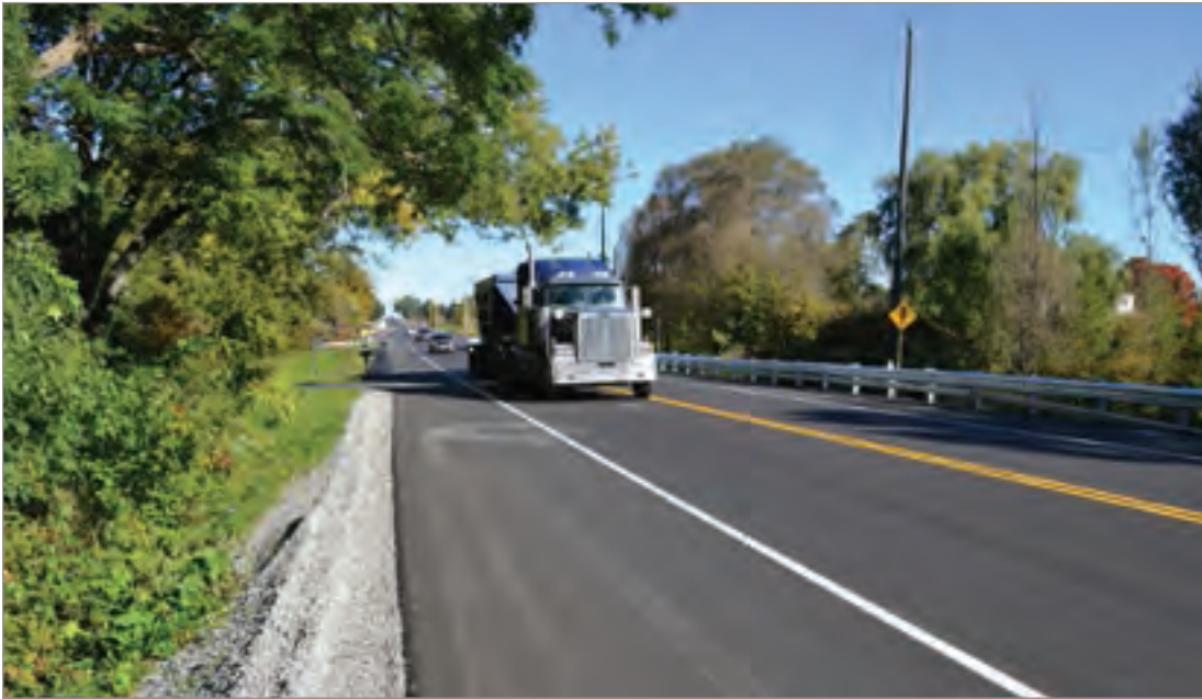
Example of a wide paved shoulder
