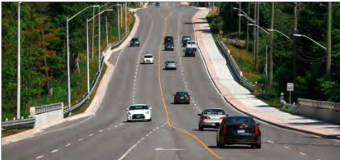
Reconstructed Warden Avenue in the City of Markham
