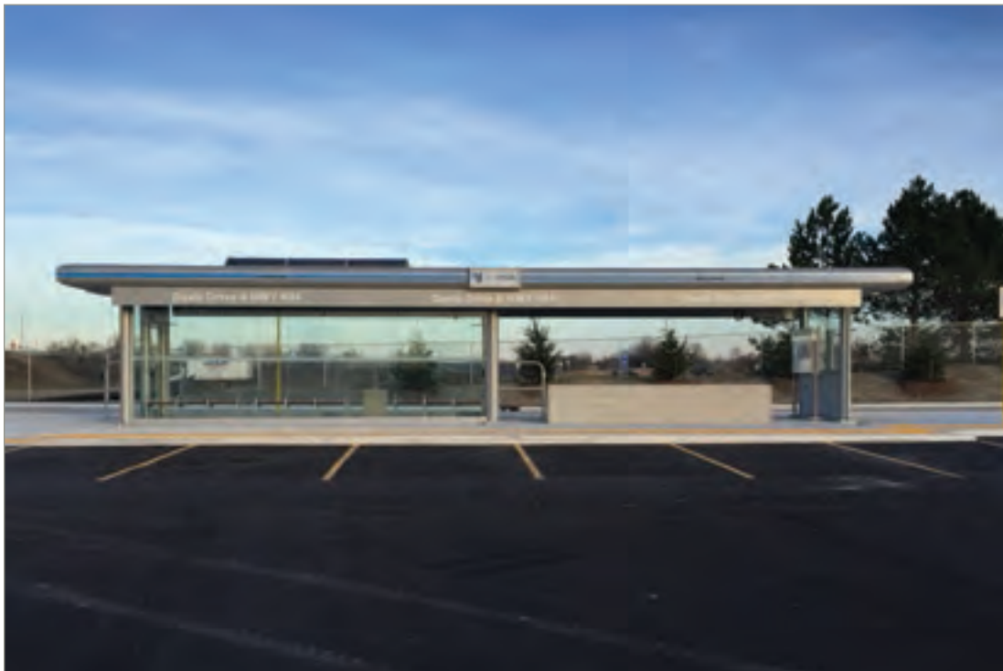
New vivastation at Davis Drive/Highway 404 carpool lot in the Town of Newmarket
