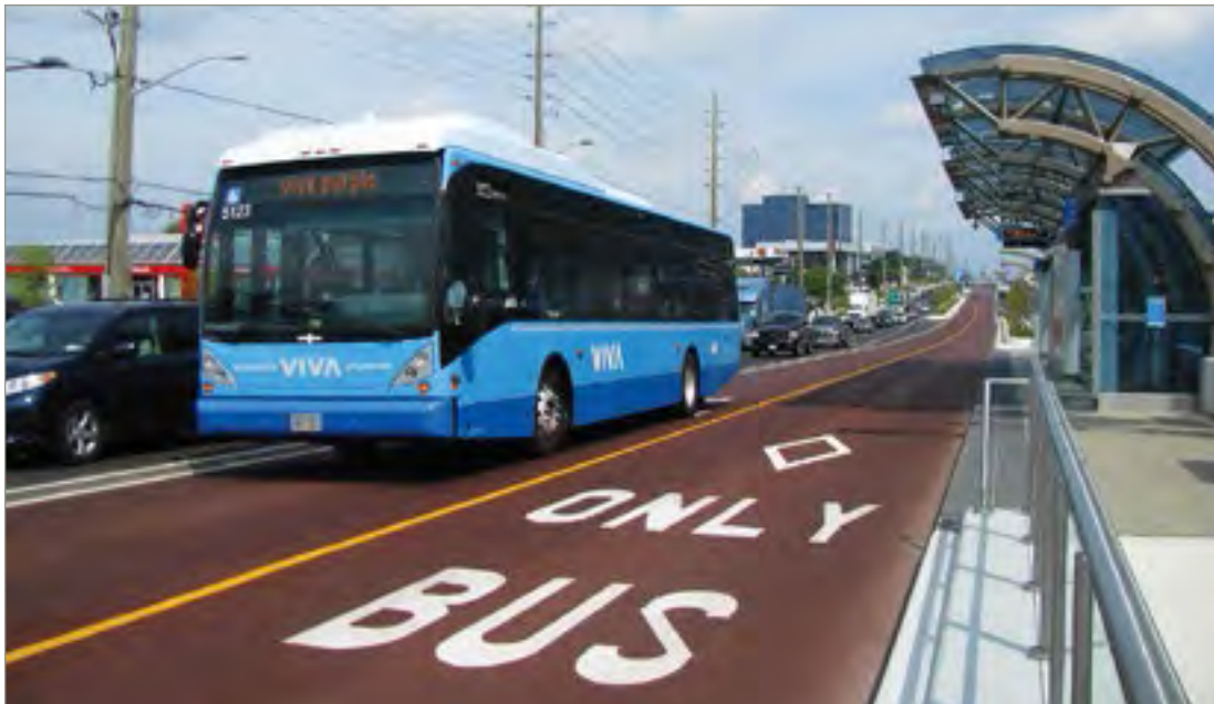
vivaNext rapidway on Highway 7, Richmond Hill
