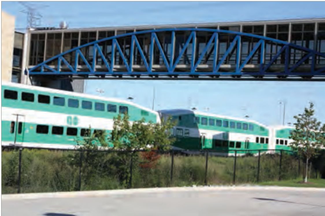
Pedestrian Bridge at the Richmond Hill Centre
