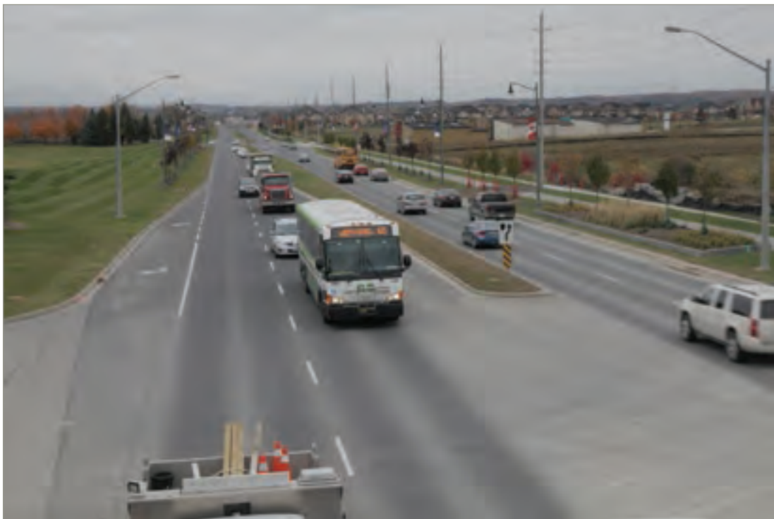
Recently re-constructed Wellington Street East in the Town of Aurora
