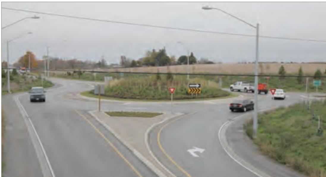
A roundabout at York-Durham Line in the Town of Whitchurch-Stouffville constructed in 2013
