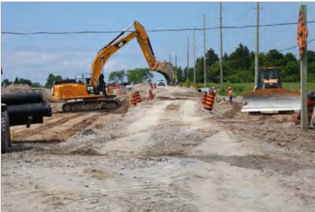
Reconstruction of 2nd Concession Road in the Town of East Gwillimbury
