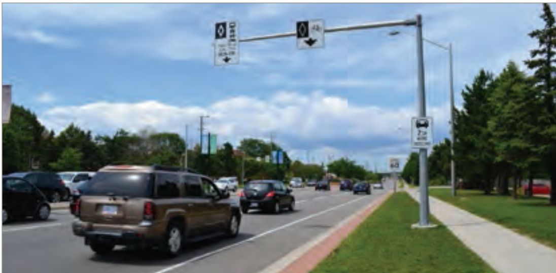
Example of HOV lanes on Dufferin Street
