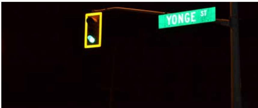
Photo: Retro reflective traffic signal backboard at the intersection of Yonge Street and Mullock Drive in the Town of Newmarket.
