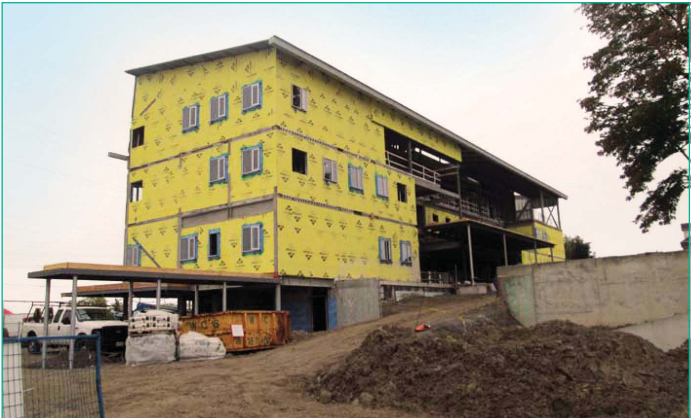
Belinda's Place construction, Town of Newmarket, November 2014
