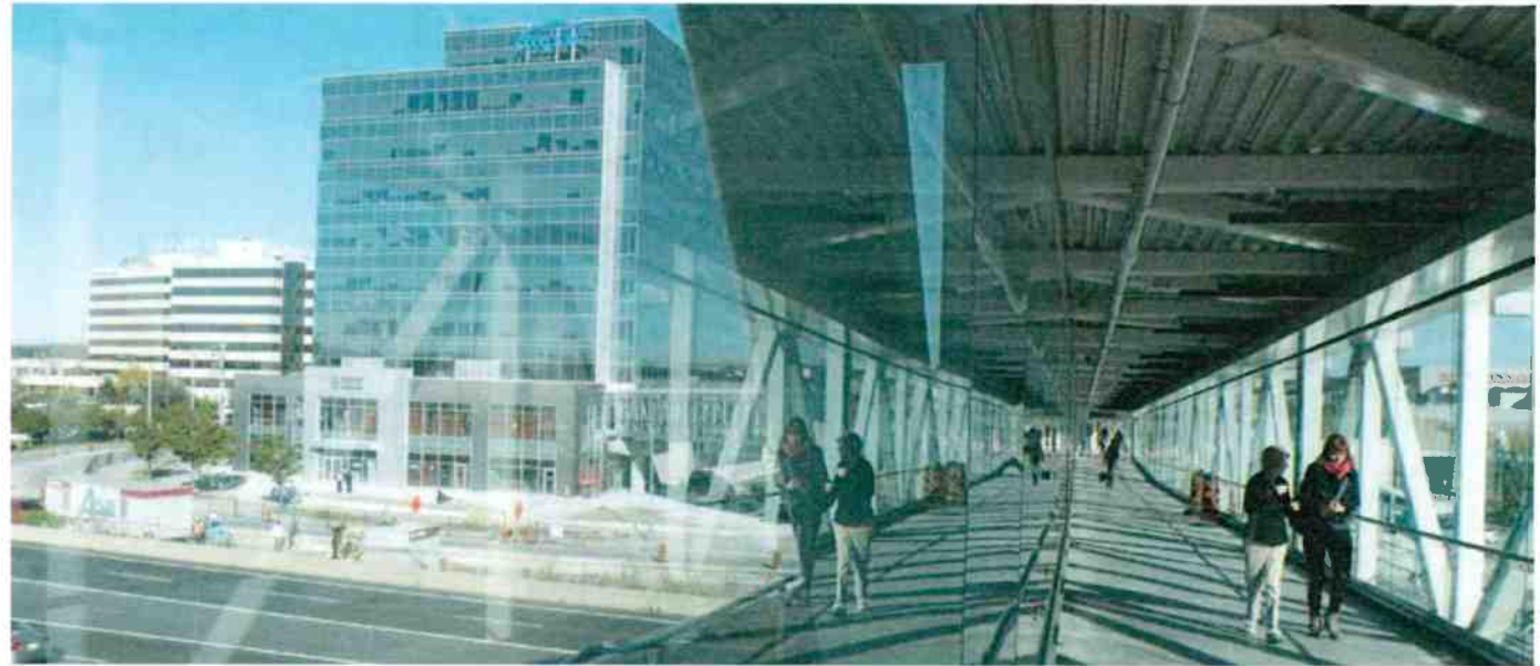
Photo courtesy of the City of Pickering
