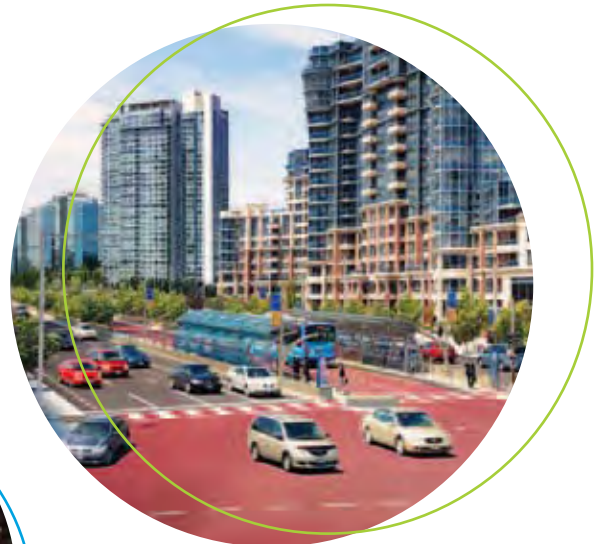
Highway 7 East Yonge Street to Warden Avenue
