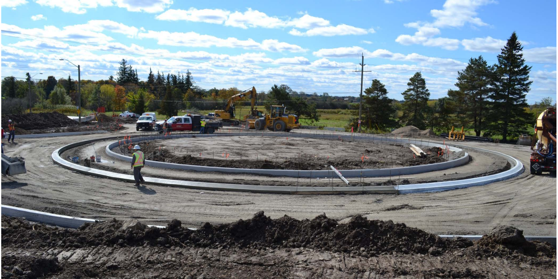
York Region's first roundabout - York Durham Line @ Durham Road 5
