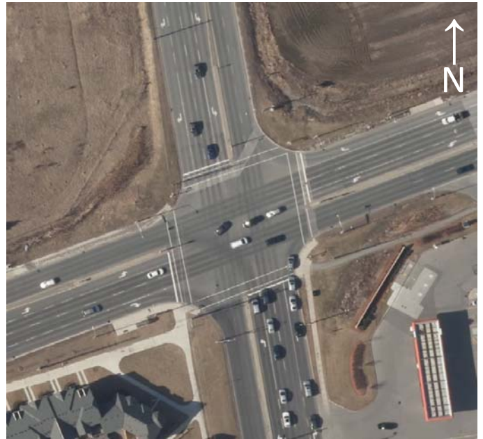
Major Mackenzie Drive at McCowan Road
