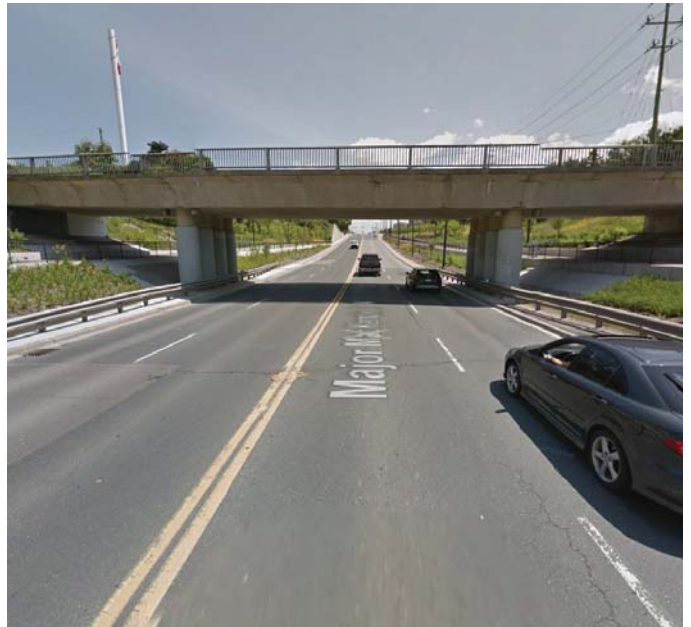
Barrie GO railway underpass east of Keele Street (Image capture: 2015, ©2016 Google)
