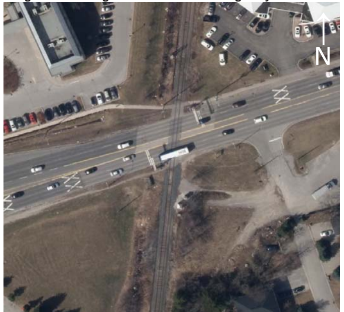
At-grade crossing of Stouffville GO at Highway 7
