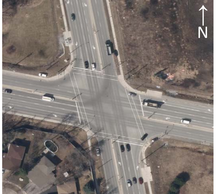
Highway 7 at Ninth Line
