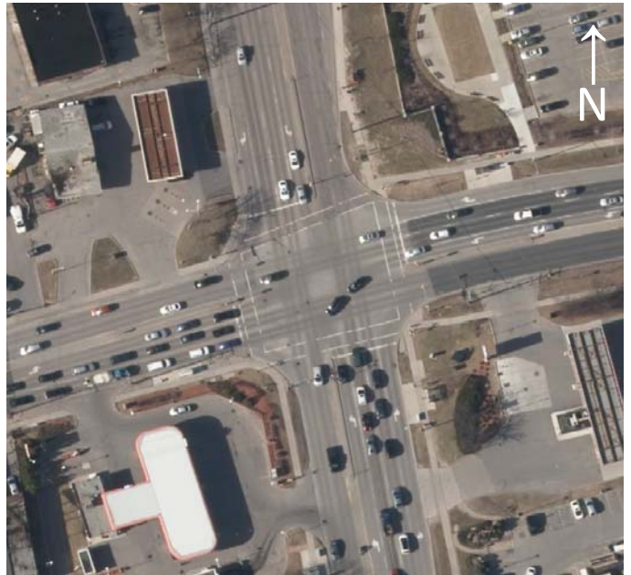
Major Mackenzie Drive at Bayview Avenue
