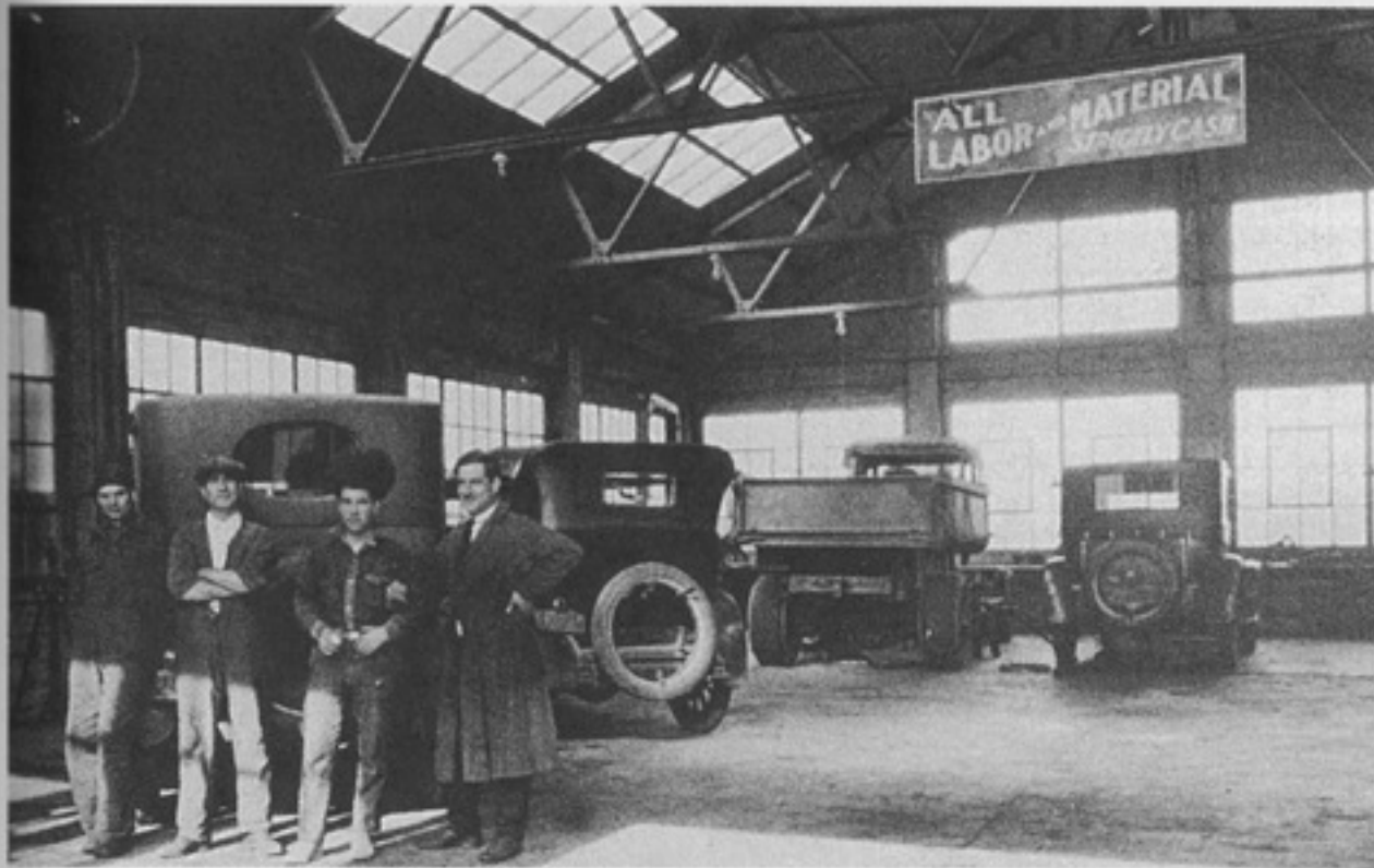
1925 - It was no doubt sometimes too cold and sometimes too hot, but the big clear-span space of the garage had the early-20th-century daylighting that is more appreciated now that it is rare. The metal roof was cheap and effective and still sounds wonderful in the rain.
