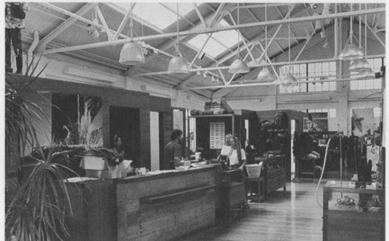
1993 - The 1924 Structure and Skin of the building was so simple and separated from everything else that it remains unchanged seventy years and many tenants later. With its abundant windows and airy steel truss overhead, it makes a cheery shop.
