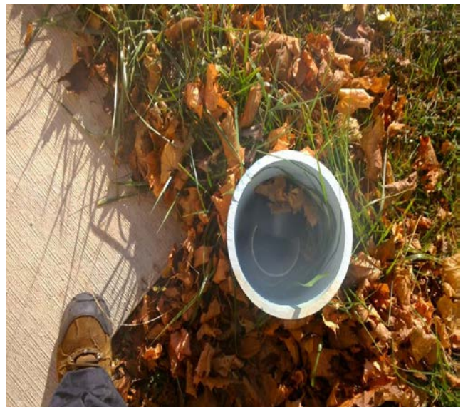
Figure 12 - Smoking Downspout and Open Sanitary Cleanout in Richmond Hill and Vaughan
