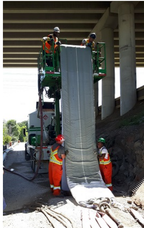
Figure 15 - CIPP liner prior to installation
