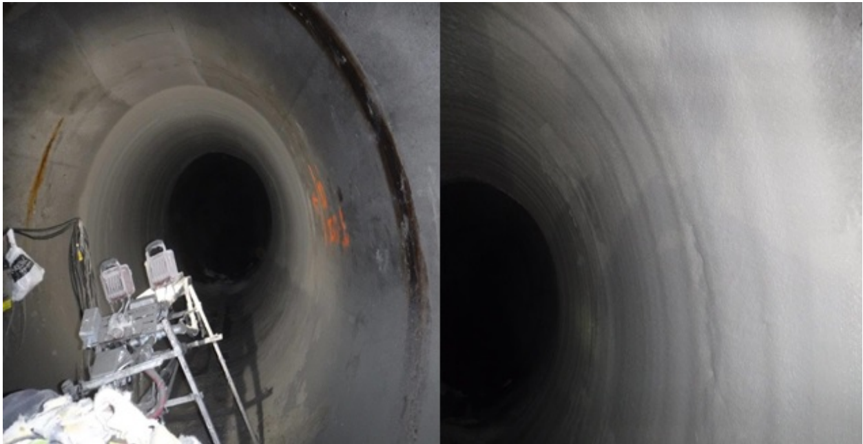
Figure 18 - 16th Avenue Trunk Sewer Gusher after Application of Geopolymer
