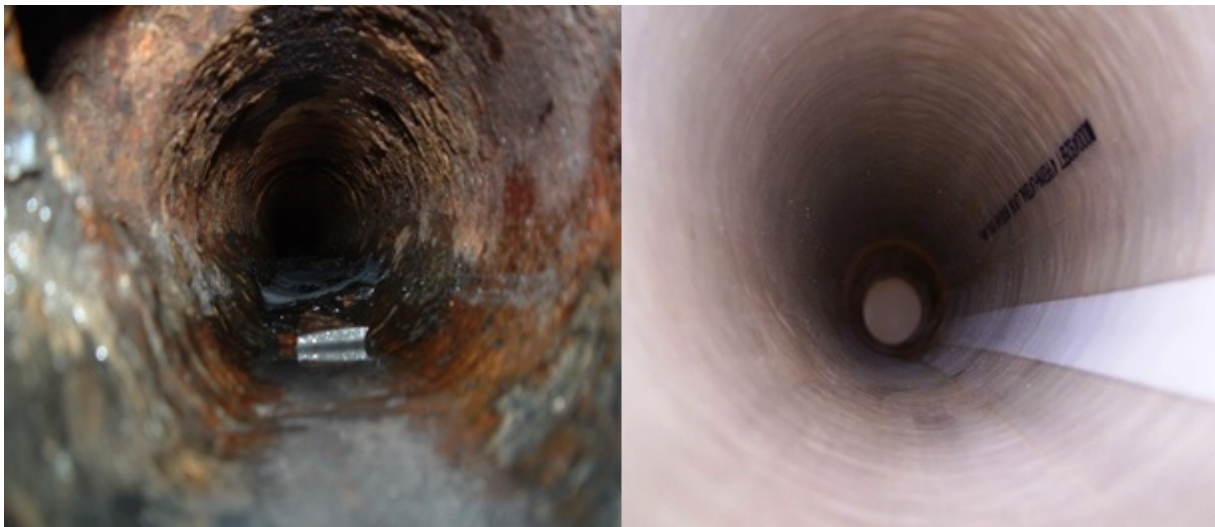
Figure 14 - Lateral Lining Before and After Rehab Illustration
